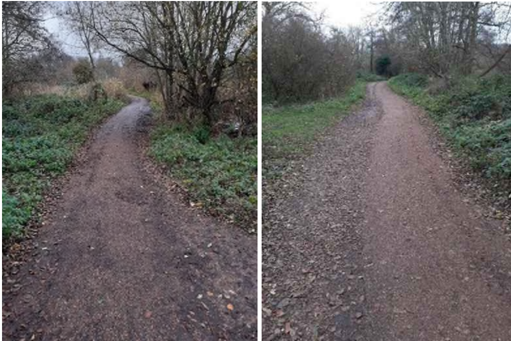
Examples of deteriorating path surface and erosion on path edges along the causeway
