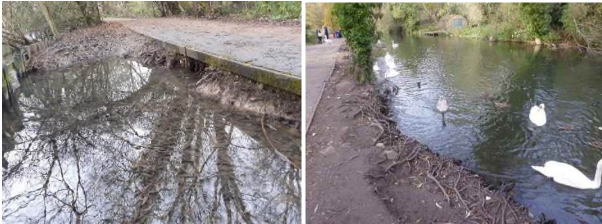
Erosion under path at northwest corner of Bury Lake; erosion and swan feeding at eastern end of Batchworth Lake
